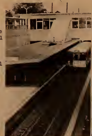
Haddonfield Station, north of Philadelphia, has similar components to the smaller new Orange Line Stations.
